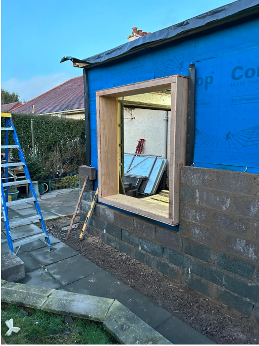
Build progress overview IMG-20260219-WA0010.jpg
