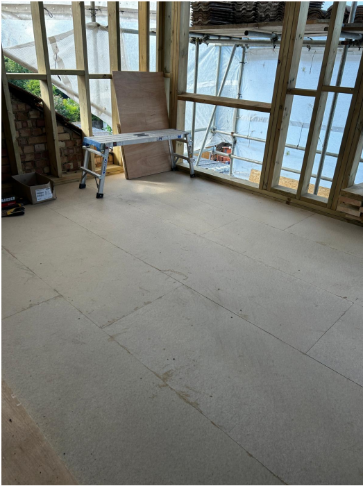
Build progress overview IMG-20260219-WA0004.jpg
