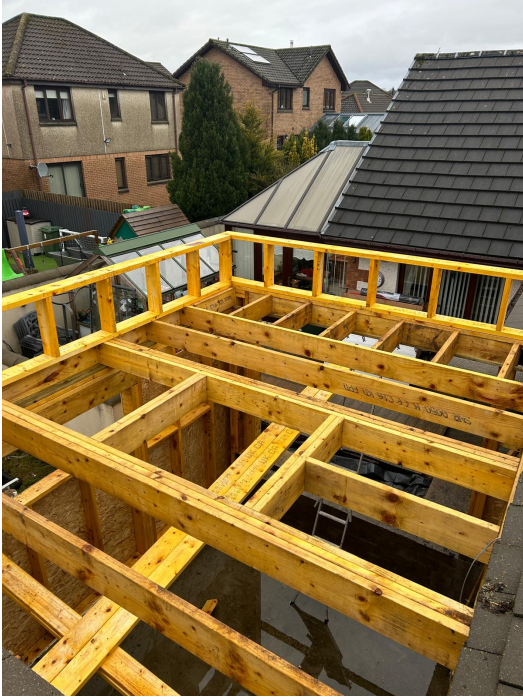
Opening-up / ceiling works IMG-20260219-WA0006.jpg
