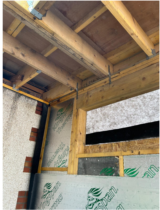
Beam / support detail IMG-20260219-WA0005.jpg
