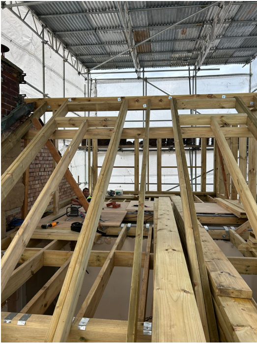
Structural timber progress IMG-20260219-WA0002.jpg
