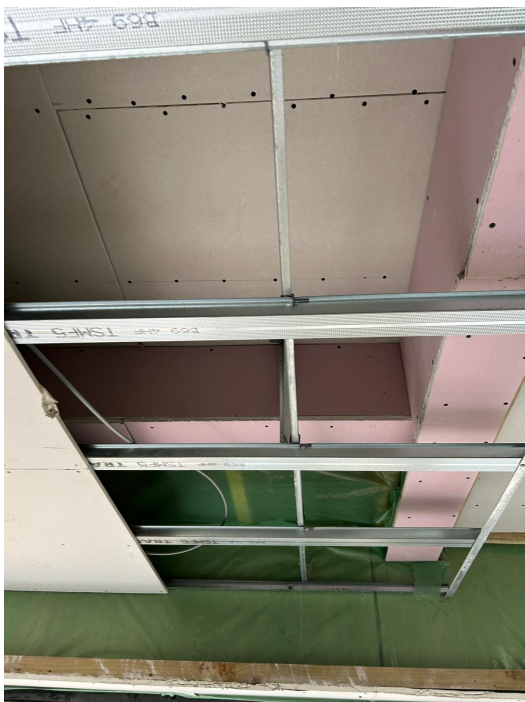
Opening-up / ceiling works IMG-20260219-WA0000.jpg
