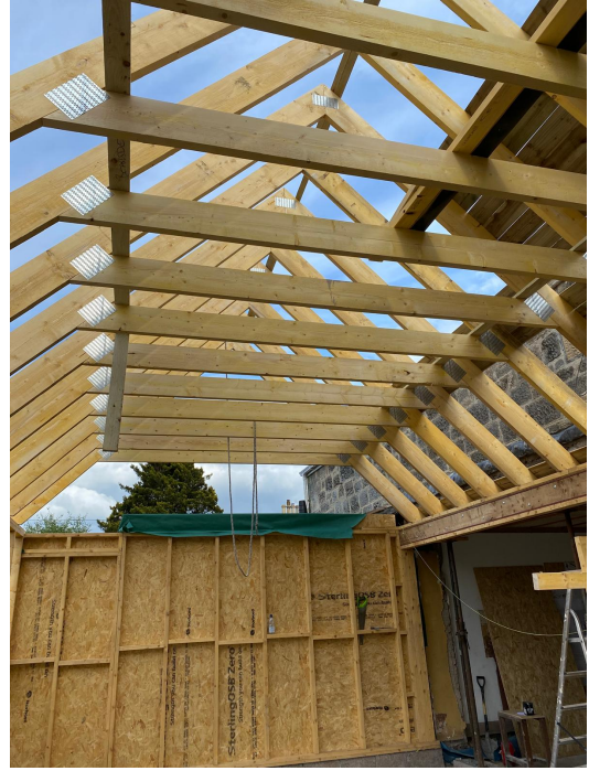
Beam / support detail IMG-20260219-WA0011.jpg
