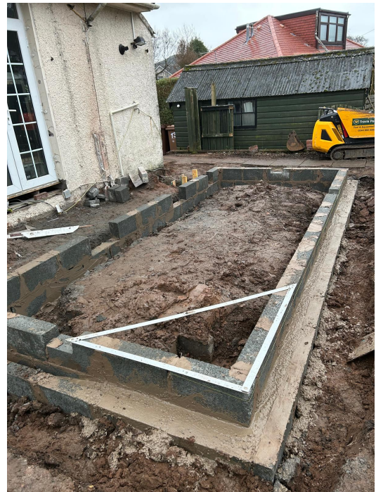
Internal framing view IMG-20260219-WA0009.jpg
