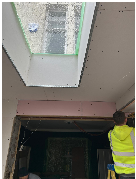
Rooflight / opening detail IMG-20260219-WA0001.jpg
