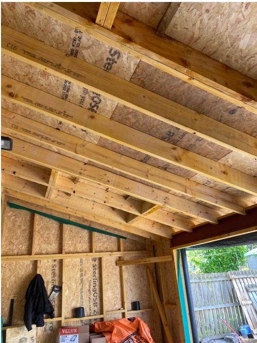
Structural timber progress IMG-20260219-WA0008.jpg
