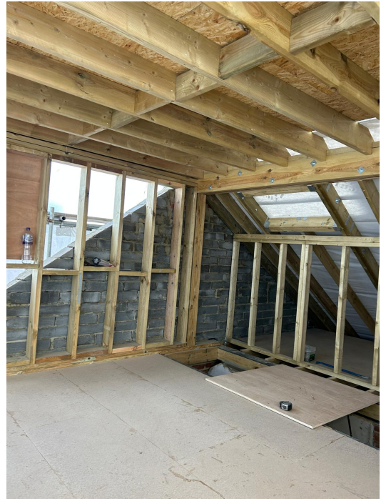
Internal framing view IMG-20260219-WA0003.jpg
