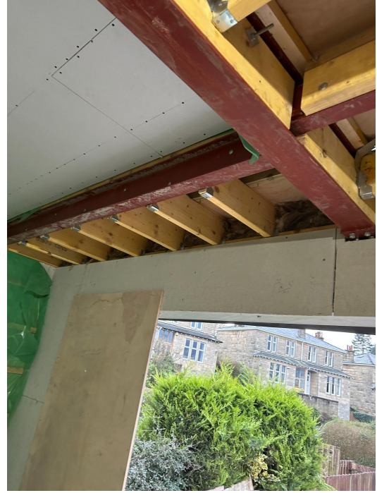
Rooflight / opening detail IMG-20260219-WA0007.jpg
