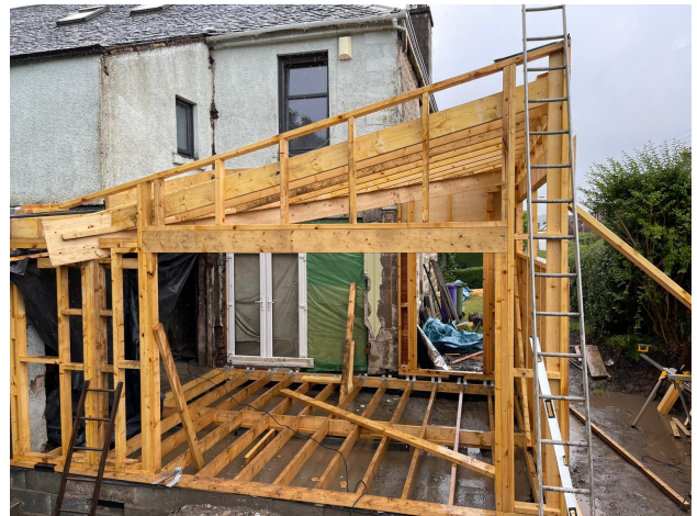
Build progress overview IMG-20260219-WA0017.jpg
