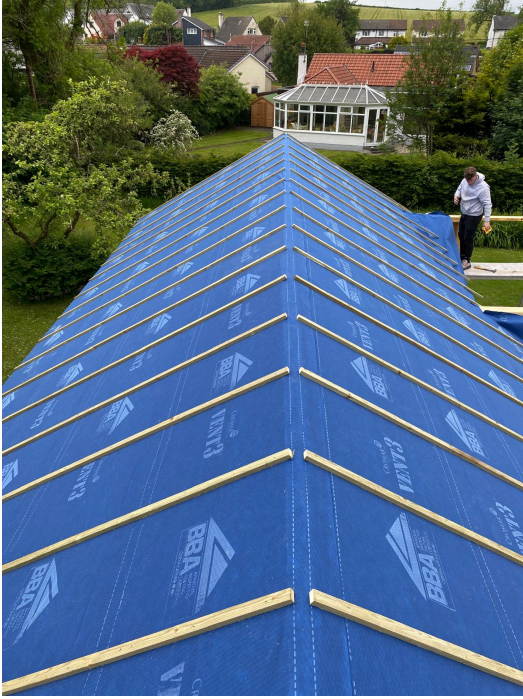
External elevation progress IMG-20260219-WA0014.jpg
