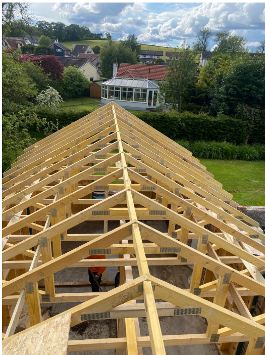
Extension framing progress IMG-20260219-WA0012.jpg
