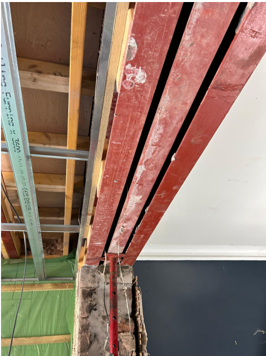
Shell construction view IMG-20260219-WA0016.jpg
