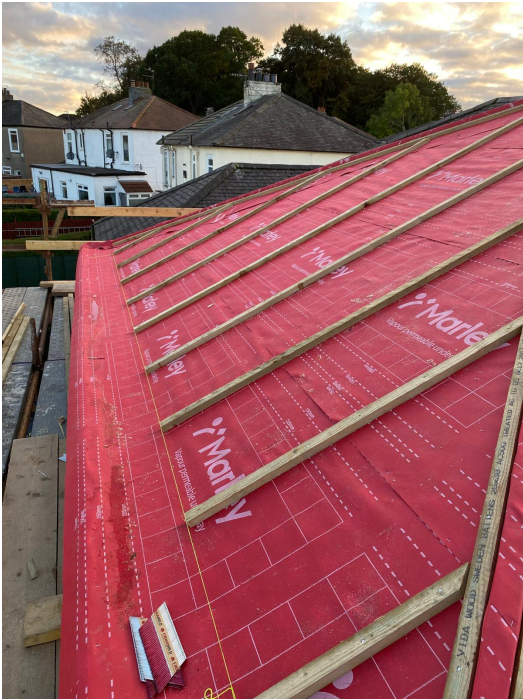
External elevation progress IMG-20260219-WA0020.jpg
