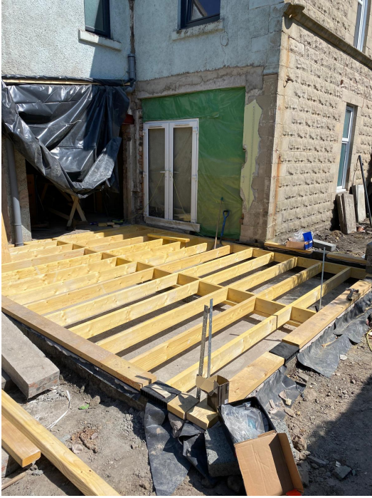
Extension framing progress IMG-20260219-WA0018.jpg
