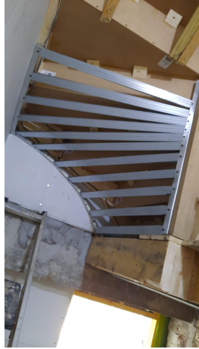
Base / formation works IMG-20260219-WA0019.jpg
