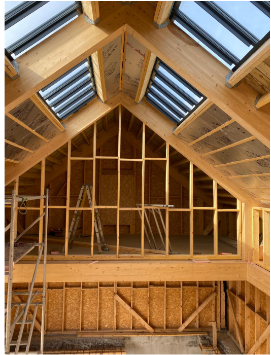
Roof framing overview IMG-20260219-WA0021.jpg
