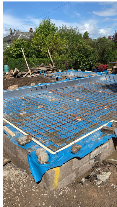
Base / formation works IMG-20260219-WA0013.jpg
