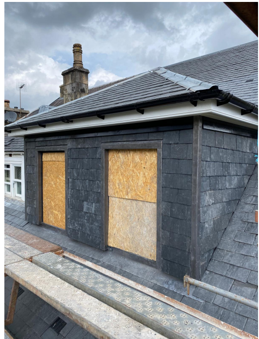
Roofline / eaves detail IMG-20260219-WA0035.jpg
