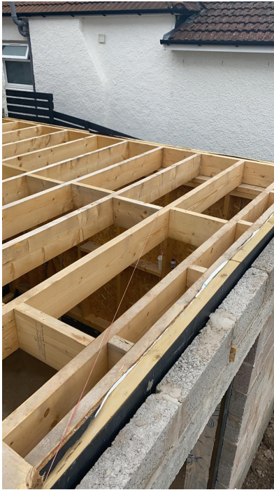
Final condition overview IMG-20260219-WA0038.jpg
