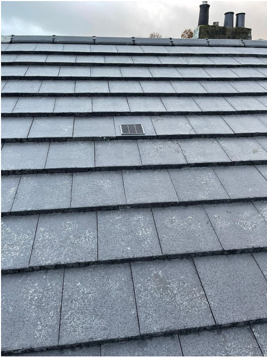
Dormer / external finishing IMG-20260219-WA0036.jpg
