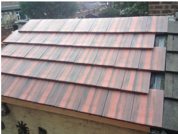
Completed roof covering IMG-20260218-WA0009.jpg
