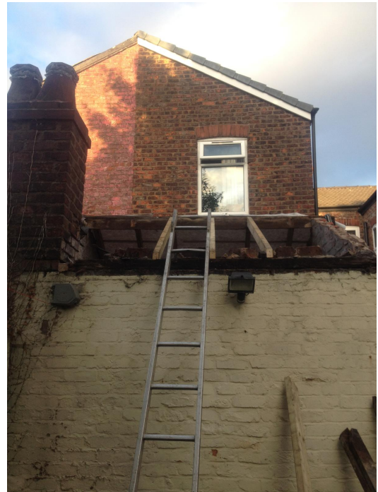
Roof replacement in progress IMG-20260218-WA0013.jpg
