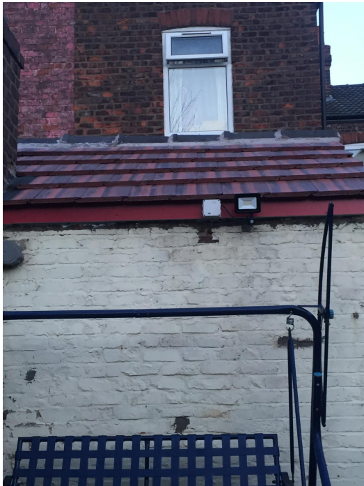
Existing roof / early stage IMG-20260218-WA0012.jpg
