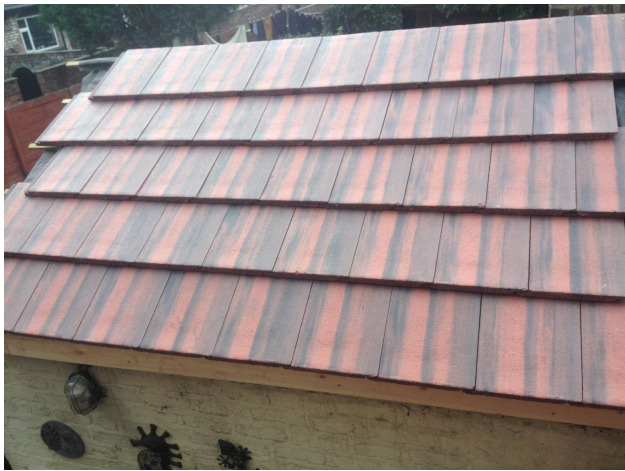
Existing roof / early stage IMG-20260218-WA0006.jpg
