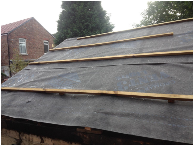
Roof replacement in progress IMG-20260218-WA0007.jpg
