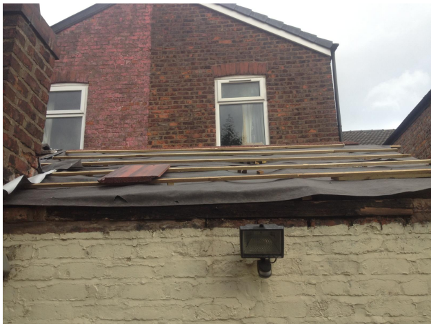
Elevation progress view IMG-20260218-WA0008.jpg
