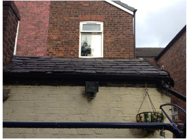
Final condition overview IMG-20260218-WA0011.jpg
